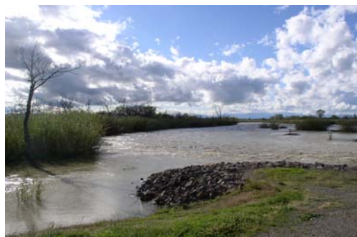
Upstream of Road P Bridge
